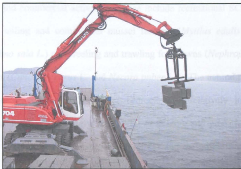
Figure 1.4. Reef module deployment. Blocks are dropped onto a target buoy from a surface barge.
