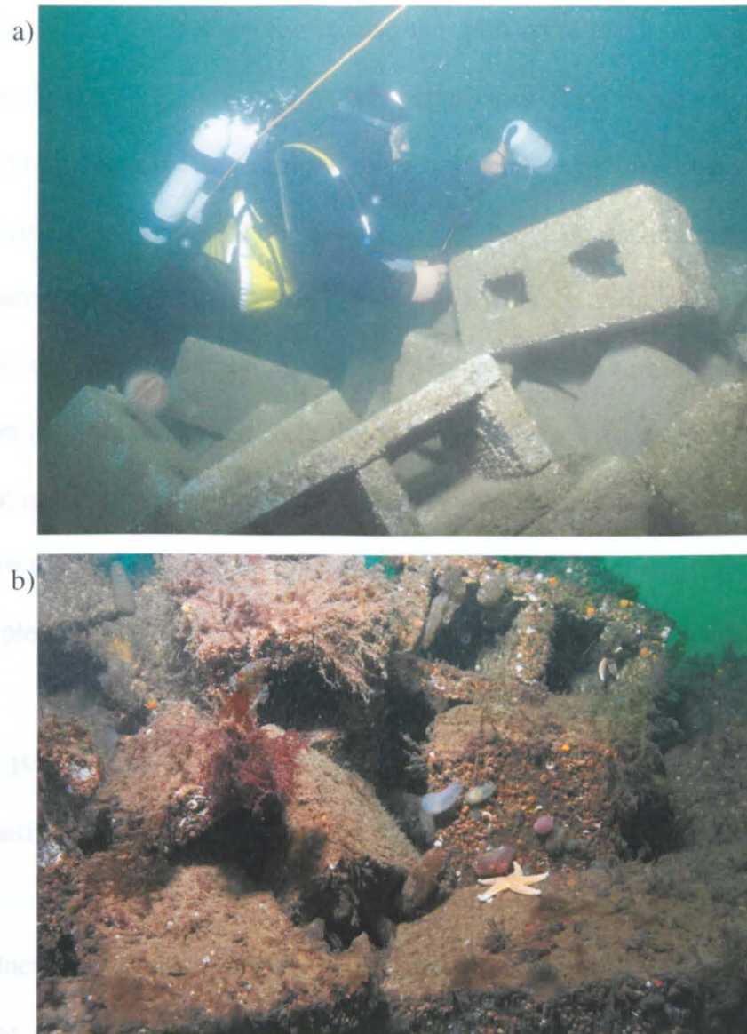
Figure 1.6. Photographs of a complex reef module within the Loch Linnhe artificial reef complex, a) shortly after deployment and b) after 2 years of fouling.
