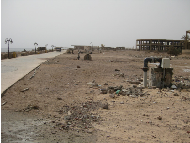
Figure 7. Well field at Dahab desalination plant
