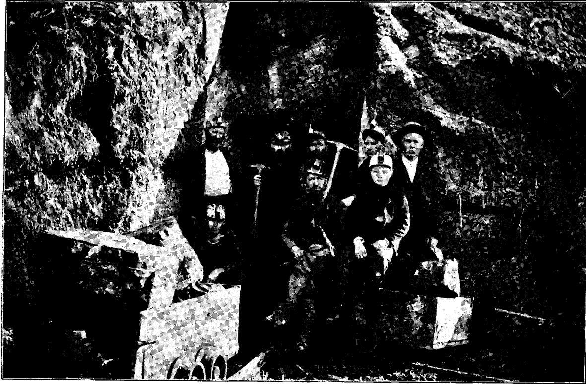
Fig. 11. The Honey Creek Coal Mine, entrance to tunnel No. 2. One of the proprietors, Mr. Hayes, stands at the right, the other, Mr. George, to the left. A group of miners stand at the entrance. To the right and left is a streak of weathered coal, which leads to a 33-inch bed near the entrance. Negative No. 8-16-2-07. Hon Charles Morrill's collection of geological photographs, the University of Nebraska.
