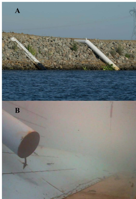
Figure 1. Images of (A) water diversion pipes located in the lower Sacramento River, California, USA and (B) green sturgeon swimming in the flume with a green sturgeon drawn (entrained) into the water diversion pipe during an experiment, recorded with an underwater camera positioned 2.1 m downstream of the pipe.
