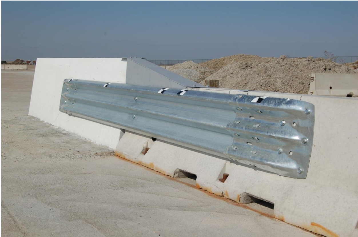
Figure 21. Free-Standing PCB to Rigid Barrier Height Transition for Median Applications on Asphalt [45]
