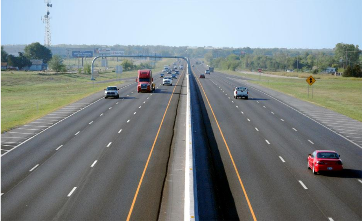
Figure 1. Double-Sided Concrete Barrier in Narrow Median [1]
