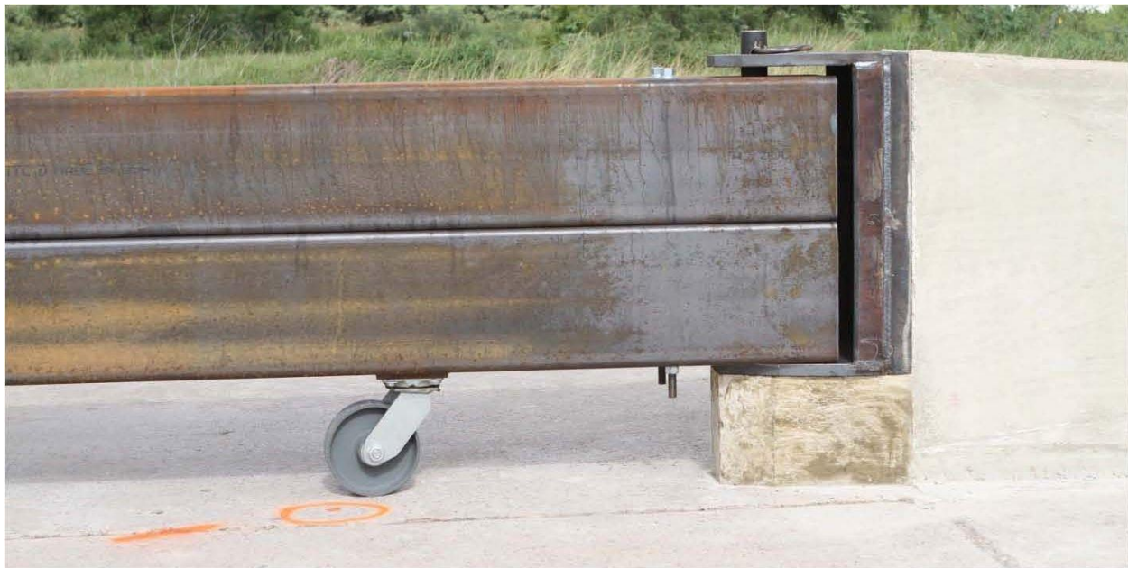
Figure 13. Final Design of the Emergency Opening System [34-35]
