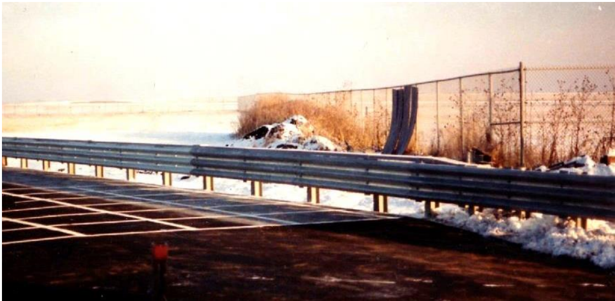
Figure 23. TBC-8000 Bridge Rail Transition [47-49]
