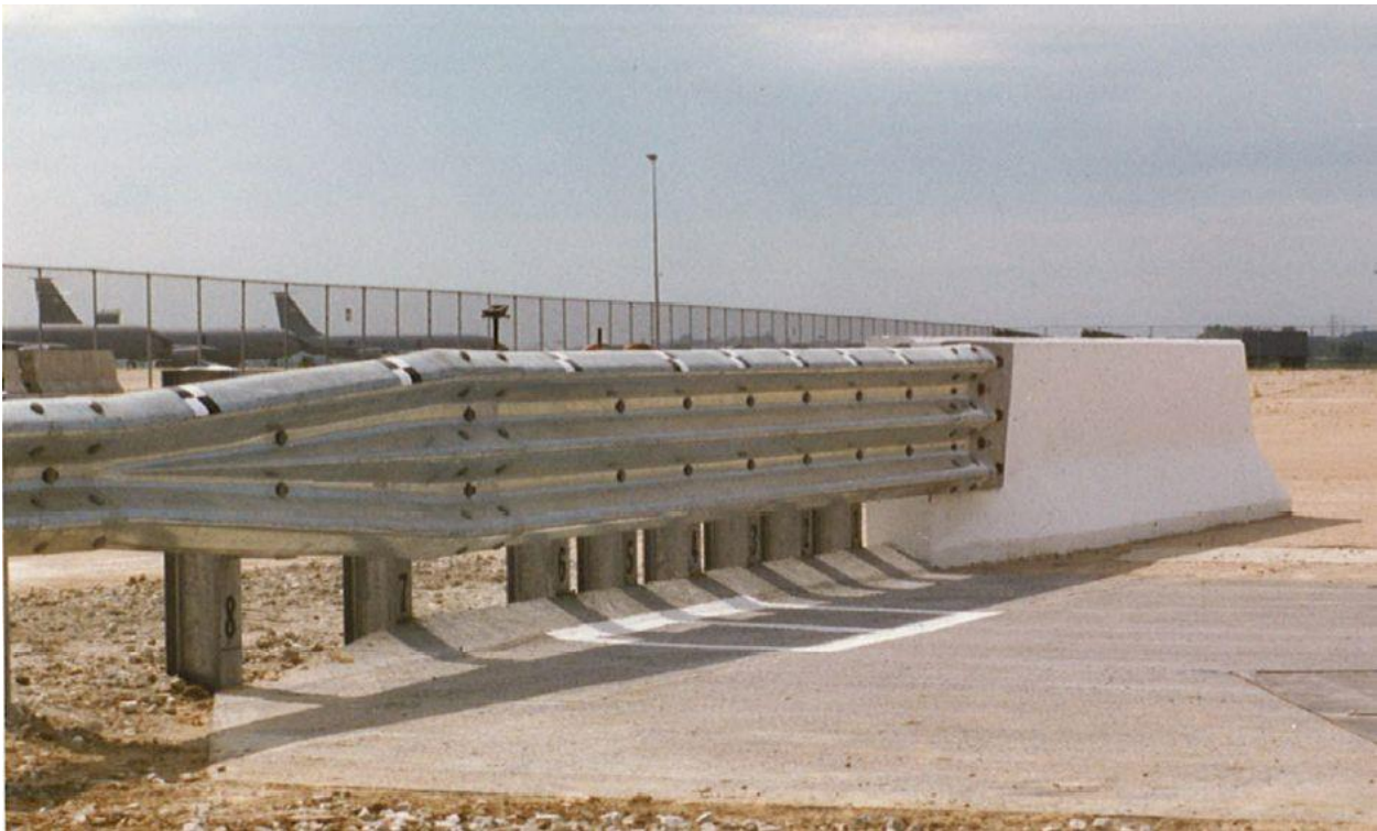
Figure 25. Horizontal Flare Rate of 6:1 Barrier Toe [53-54]
