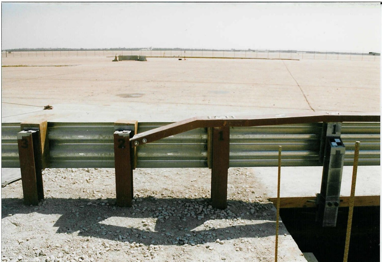
Figure 24. TL-4 Transition on Transverse Glue-Laminated Timber Deck [51-52]
