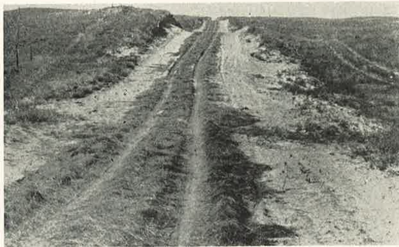
FIGURE 12.—A graded, sandhill road of Thomas County, held against wind erosion by a spread of hay and weeds.
