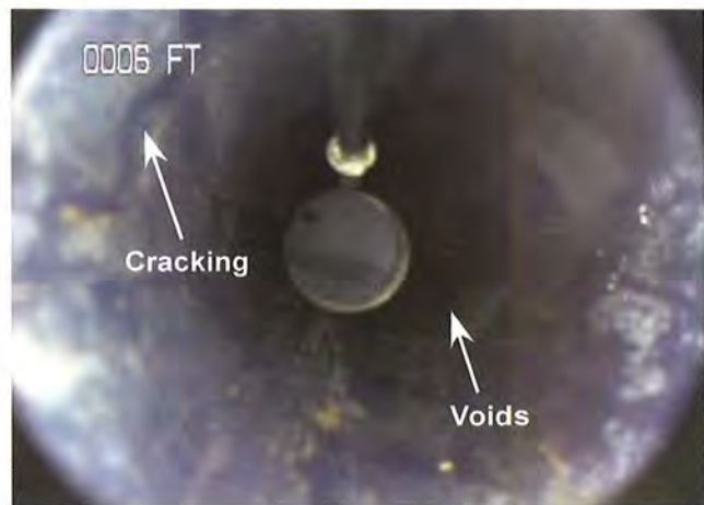
Figure 24. Cracking and voids in the Trenton bentonite slurry.
