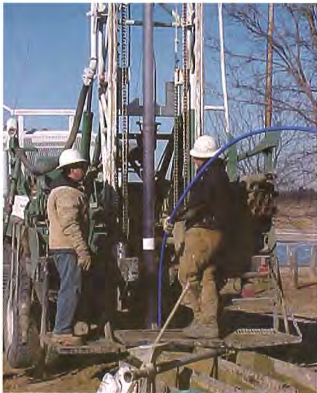
Figure 3. Installation of clear PVC casing with tremie pipe.
