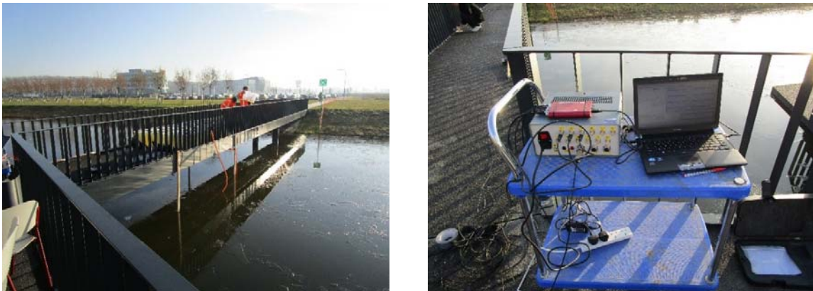
Fig. 1: Bridge 1 – left: side view and right: data acquisition station
