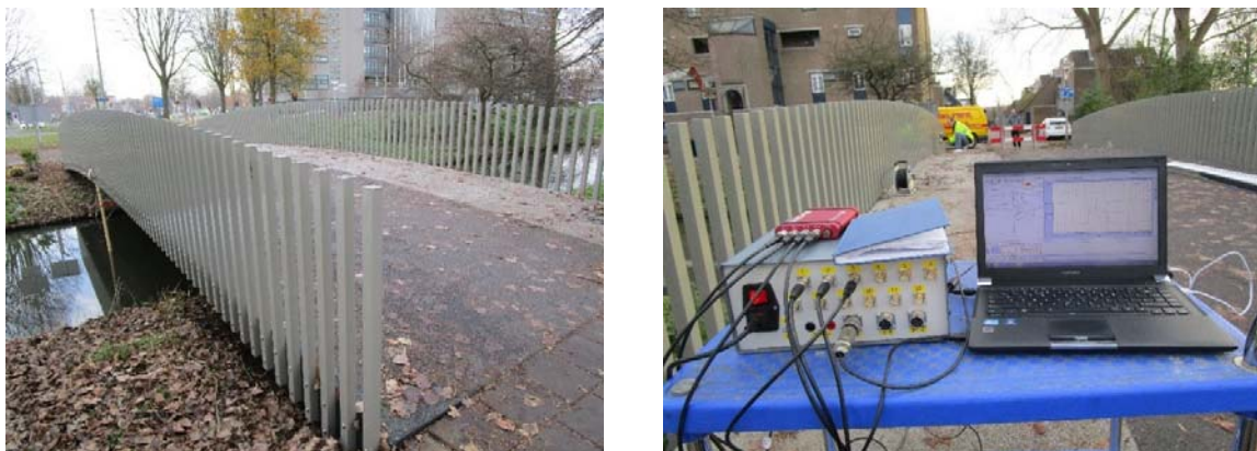
Fig. 2: Bridge 2 – left: side view and right: data acquisition station
