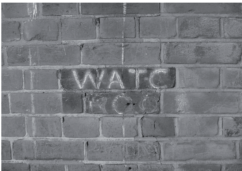
Figure 1. WATCH ROOM: painted sign on the wall of a school building.
