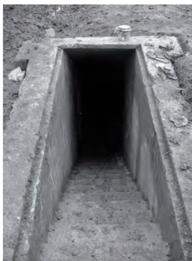
Figure 2. The entrance of the shelter, following excavation.
