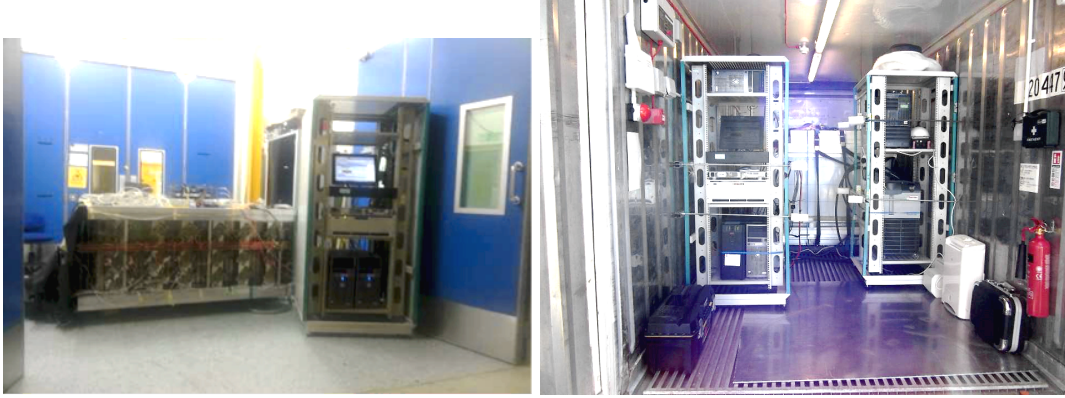
Figure 1: Pictures of the completed anti-neutrino detector. Left: at Liverpool. Right: Installed into the shipping container.
