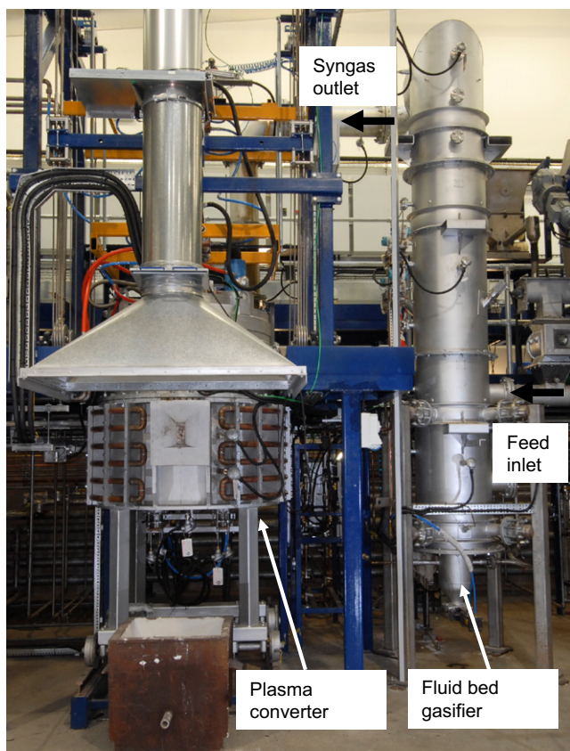
Fig. 3. APP demonstration plant.
