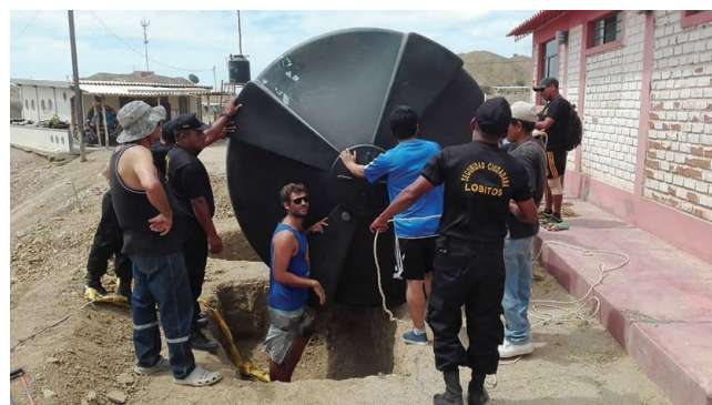
Figure 4. Installation of biodigester at the Lobitos FG
