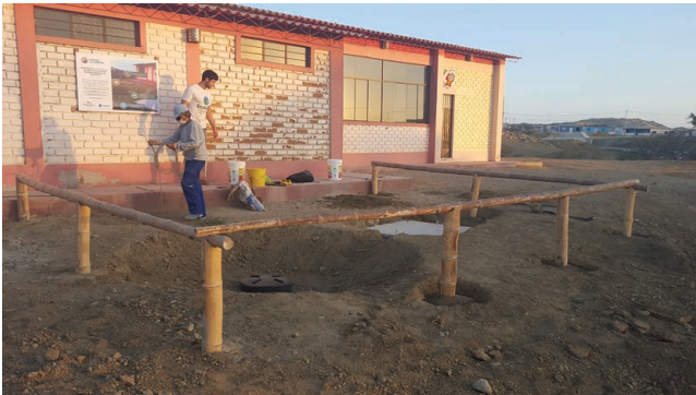
Figure 6. Completed installation of biodigester with fencing protection
