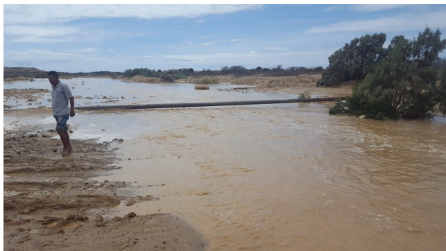
Figure 3. Flooding damages key water pipeline into Lobitos in 2017
