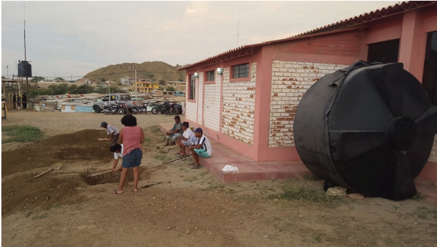
Figure 5. Installation of biodigester at the Lobitos FG
