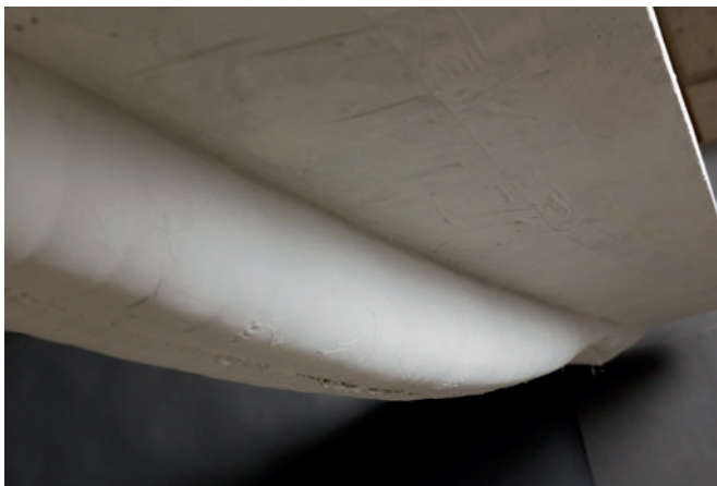
Fig. 7: Flexibly formed concrete beam.
