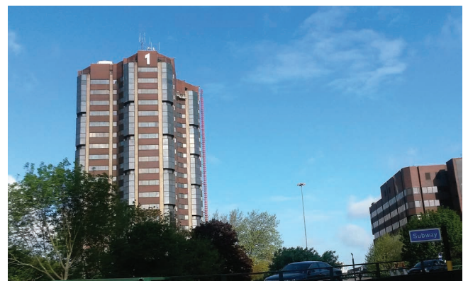
Figure 5. One Hagley Road during internal construction work
