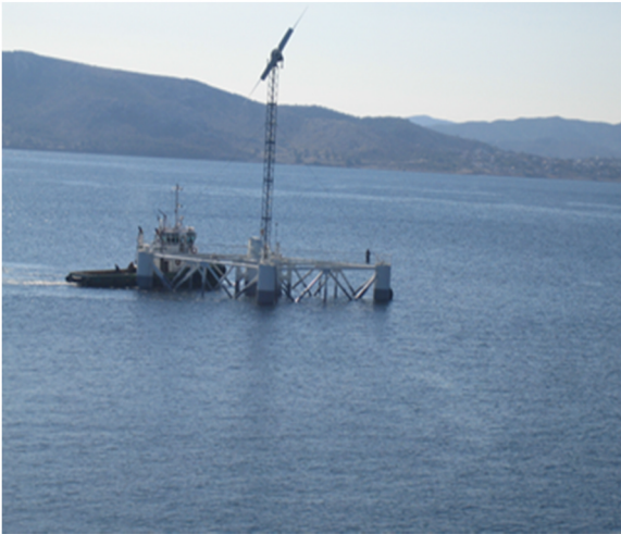
Fig. 9. Ydiada platform with 35 kW wind turbine in Heraclea (image permission from Ecowindwater).
