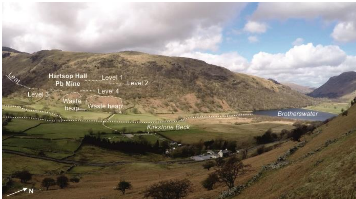
Fig. 2 The view west across the floodplain of Brotherswater highlighting the location of Hartsop Hall mining infrastructure, shaft levels, exposed waste heaps and their proximity to the river. The levels were sunk incrementally, with the first ore extracted from level 1 and shafts 3 and 4 dug during peak mining in the 1860s and 1870s. A colour version is available online.
