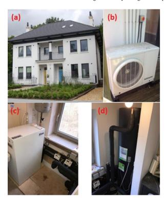
Fig. 2 (a) Building Research Establishment (BRE) Natural House, (b) Glen Dimplex heat pump, (c) Glen Dimplex Quantum Boiler, (d) Hot water storage tank
