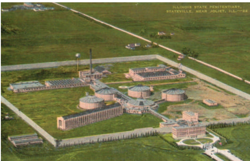
Figure 2: Stateville Penitentiary, near Joliet, Illinois, 1916-24, architect W. Carby Zimmerman. From a 1930s postcard reproduced at www.people.fas.harvard.edu/~wellerst/collection/
