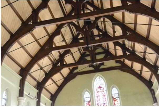
St Gerard's Church (1908), Wellington - King-post truss
