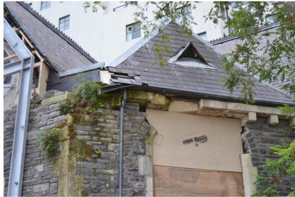
(d) Interactions between nave and its roof - Trinity Congregational, Central Christchurch
