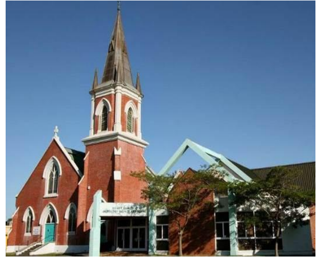
(b) Wesley Broadway Methodist Church (1911), Palmerston North - Presence of adjacent buildings and raised element
