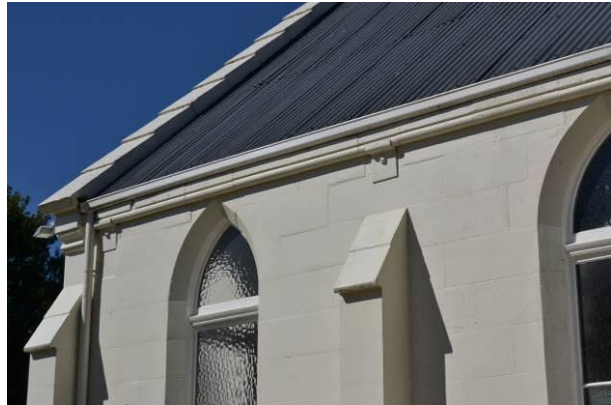
(b) St Magnus (1897), Duntroon - Tie rods connecting walls
