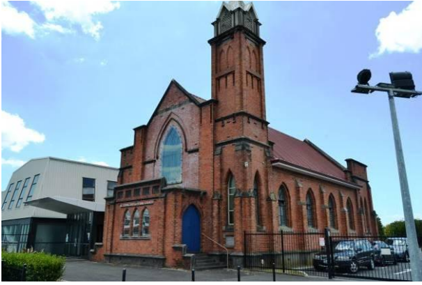
(a) St John's (1922), Auckland - Porch facing the façade
