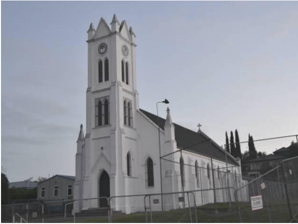
(a) St Mary's (1888), Pleasant Point - Bell tower included in the façade
