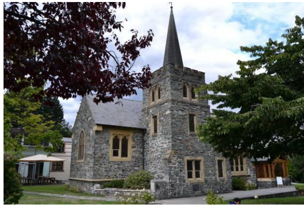
(c) St Peter's (1932), Queenstown - Bell tower along the longitudinal walls
