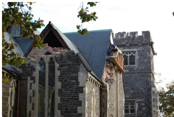
(c) St Peter's Church (1875), Christchurch (Photo courtesy of Joao Leite) - Two-layer wall
