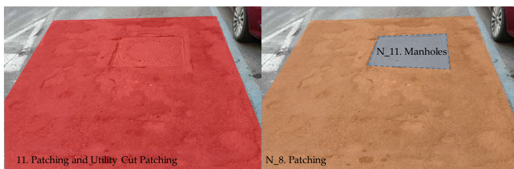
Figure 3-8. Example of manhole distress identification guidelines, Manholes
