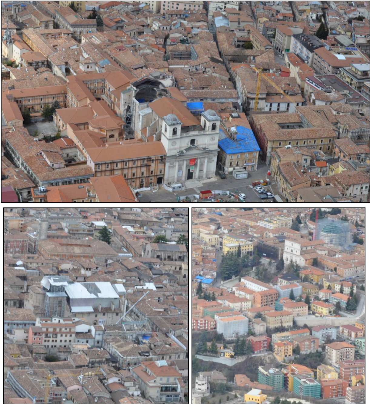
Figure 3. Various examples of collapse of the church roofs (which continue to show evident openings), temporary patching and covering of the roofs, thick wrapping works and presence of cranes in L'Aquila. Photos: Geographical Unit (Department of Documentary, Linguistic-Philological and Geographical Sciences) of the Sapienza University of Rome (in collaboration with GREAL, European University of Rome) (March 2012).
