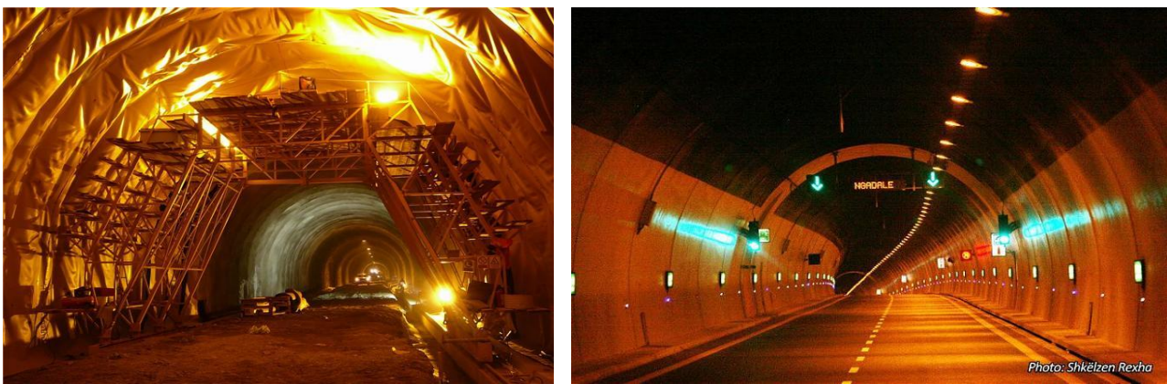
Figure 4.11 Thirr Tunnel, Milot- Morine section
