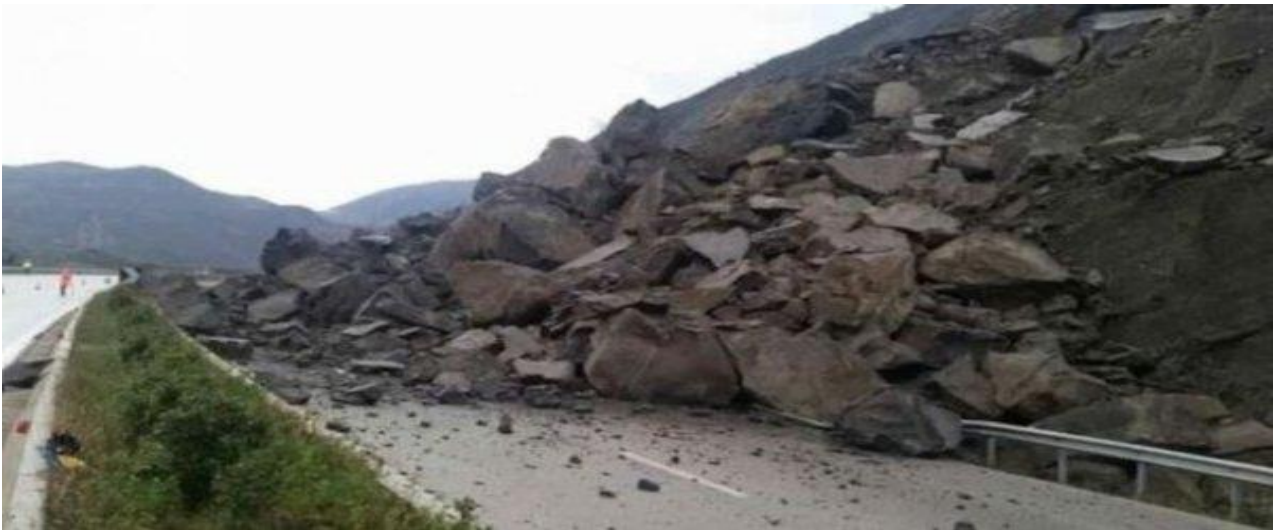
Figure 4.12 Falling stones, Rreshen- Morine section
