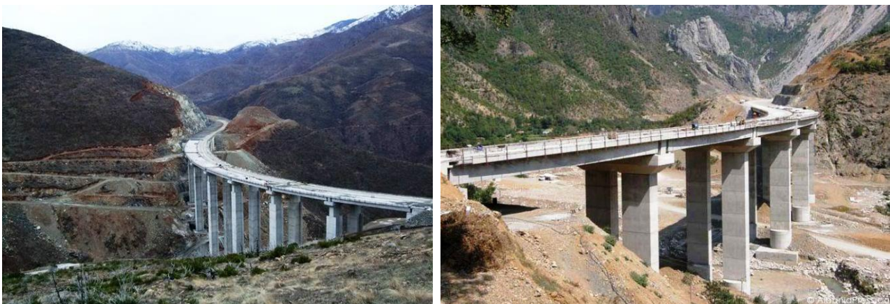
Figure 4.10 Bridges of Milot- Morine section
