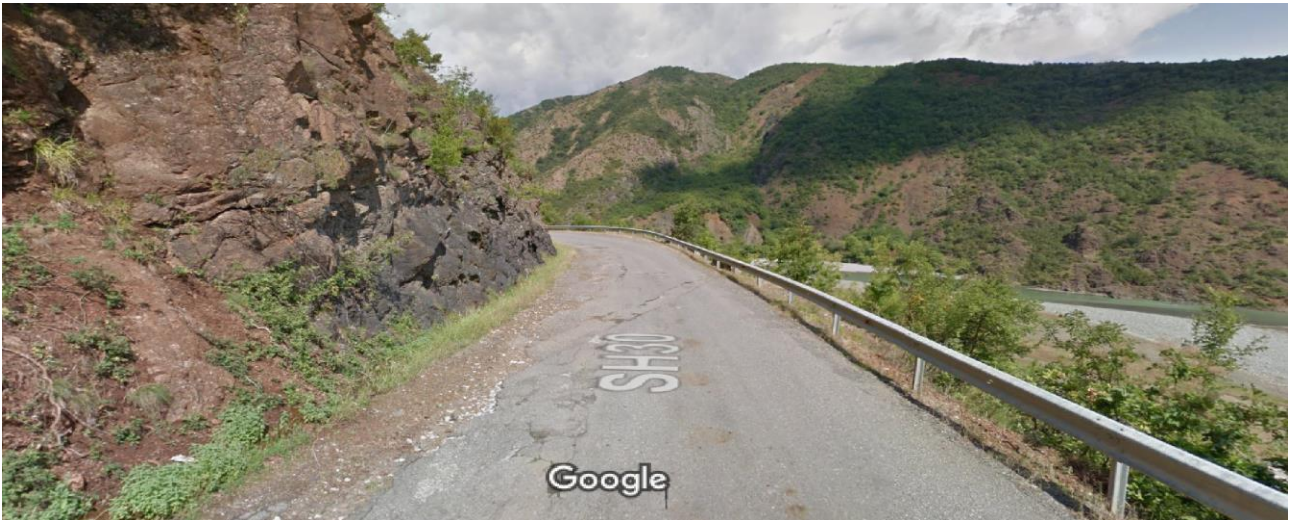
Figure 4.15 Secondary road connecting the highway to the city of Rreshen
