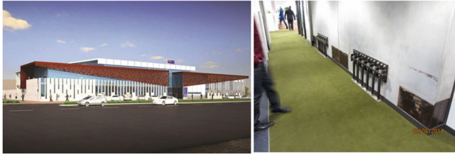
Fig. 13.26 Police Station in Rotorua. Post-tensioned concrete (PRESSS) walls with external & replaceable dissipaters in both directions (Structural Engineers: Spiire)
