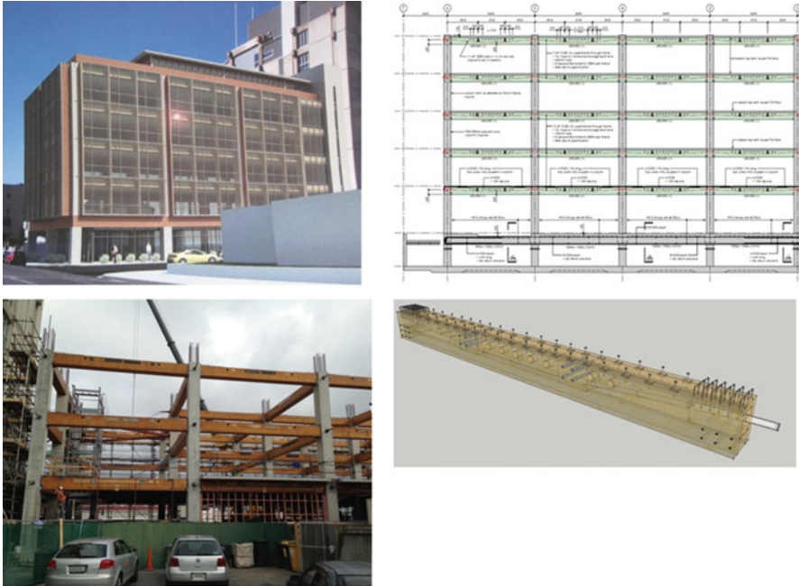
Fig. 13.33 Former ‘St Elmo Courts’ Building, Christchurch. Five storey building, combining base-isolation and two-ways post-tensioned frames in the superstructure with timber beams and concrete columns (Architect: Ricky Proko, Structural Engineers: Ruamoko Solutions)
