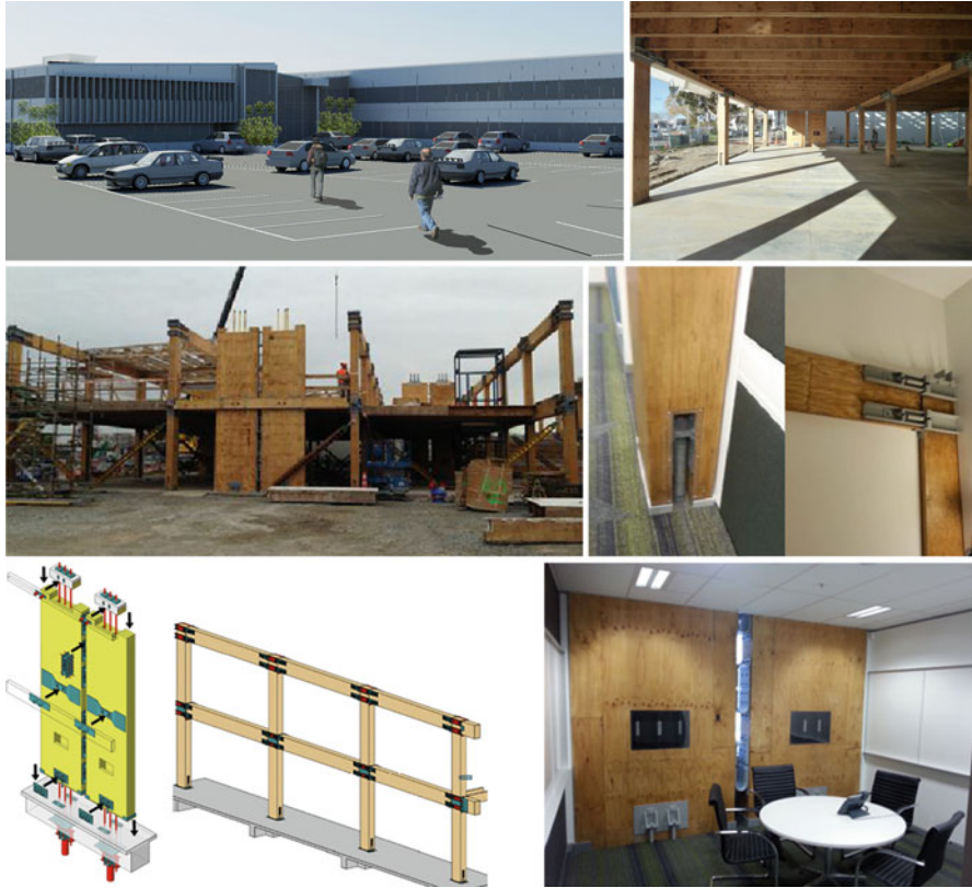
Fig. 13.32 Trimble Building , Christchurch. Two storey office building (more than 5,000 m 2 ) consisting of post-tensioned timber (Pres-Lam) frames with external replaceable dissipaters at the beam-column connections and at the column-to-foundation connection and Pres-Lam coupled (with UFP, U-shape Flexural Plates) walls with external dissipaters at the base-connections (Design-build project with Architecture and Structures by Opus International and construction by Mainzeal/City Care, Brown et al. 2012)
