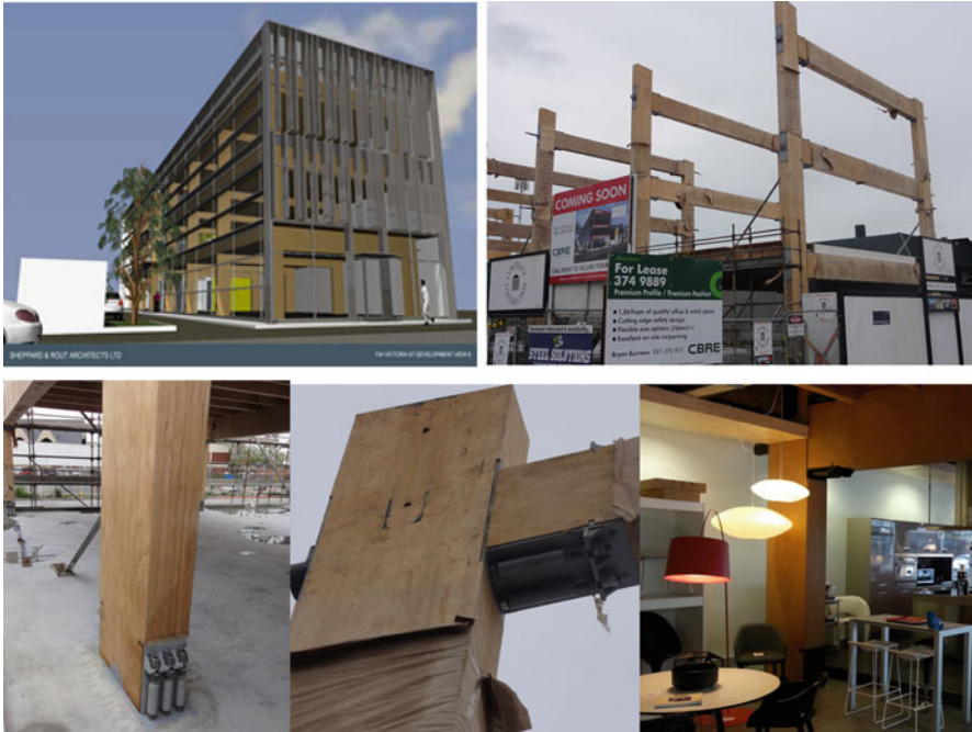
Fig. 13.31 Merritt Building, Victoria Street, Christchurch. Three Storey commercial Building consisting of Post-tensioned timber (Pres-Lam) frames in the transverse direction and cast-in-situ reinforced concrete wall in the longitudinal direction (Structural Engineers: Kirk and Roberts; Architects: Sheppard and Rout)
