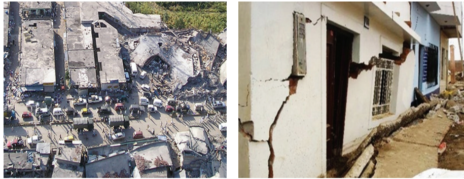
FIGURE 5: Damage of earthquake in Pakistan.
