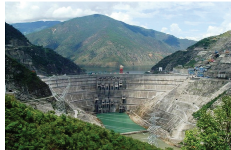
FIGURE 2: Downstream elevation of the arch dam.
