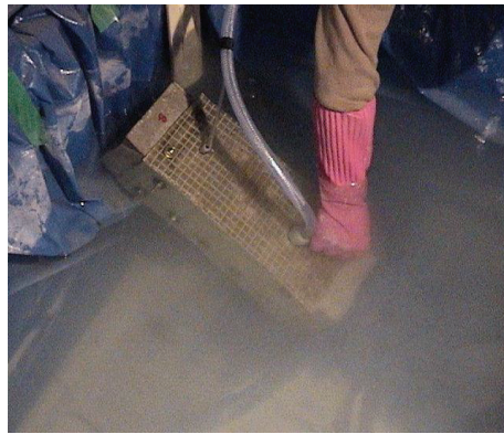
(f) Injection of repair materials
