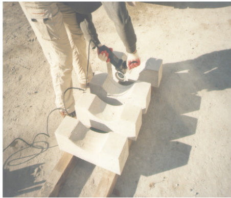
(c) Chipping of concrete
