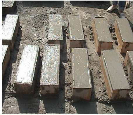
(a) Forms after pouring concrete
