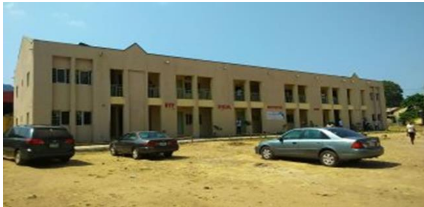
Figure A6: Picture of the north façade
