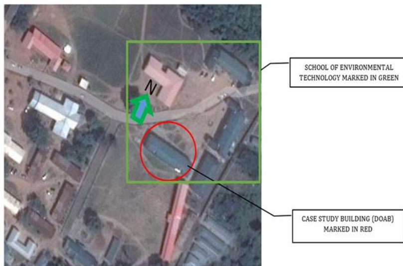
Figure 6: Aerial view of the case study building (DAOB). (Source: Adopted from Google Earth, 2015).
