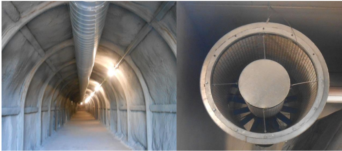
a) Tunnel and fan duct
