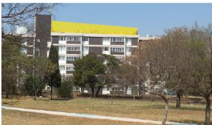
5: Alexander Rd, Roof top
