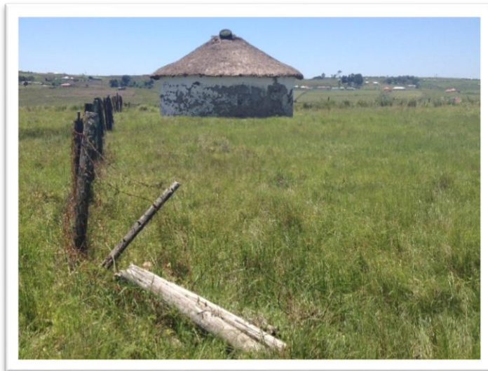
Lindiwe’s first school classroom, now derelict
