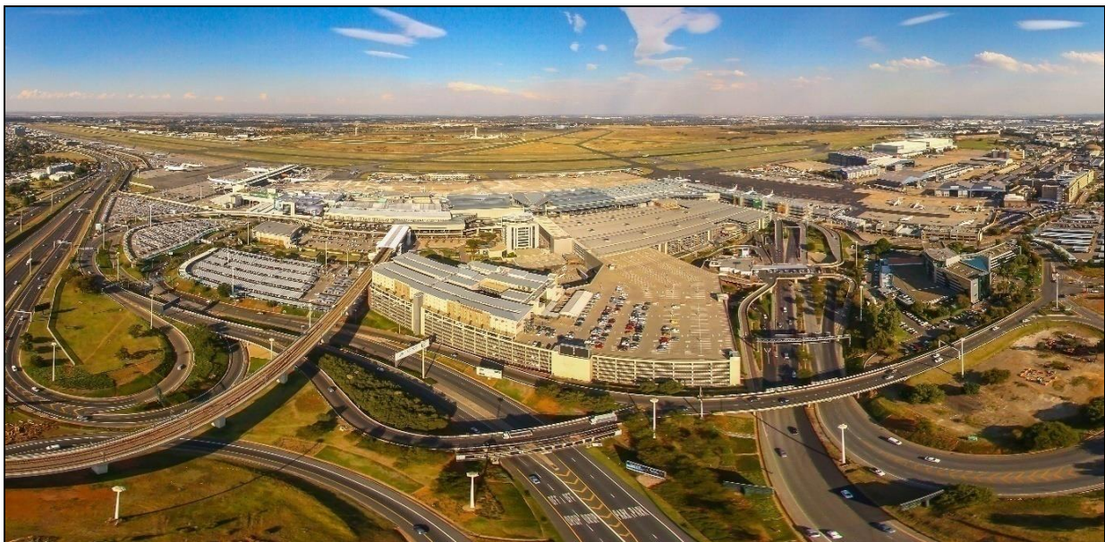
Figure 6- Aerial View of O.R Tambo International Airport
