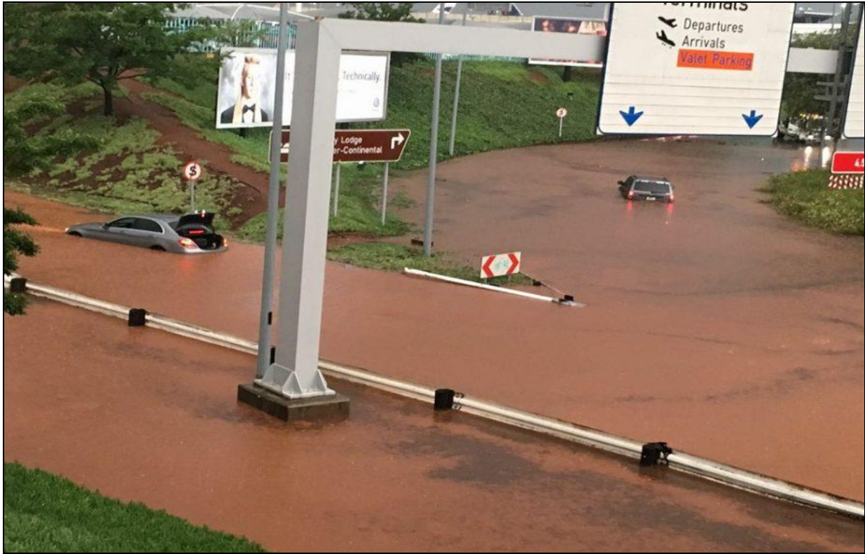
Figure 20- ORTIA Flooded After Heavy Rains
