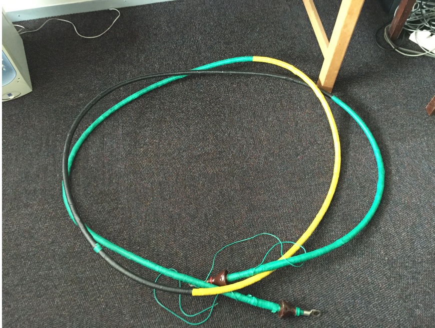
Figure 4.3: 8.25 m 11 kV single core cable used in testing
