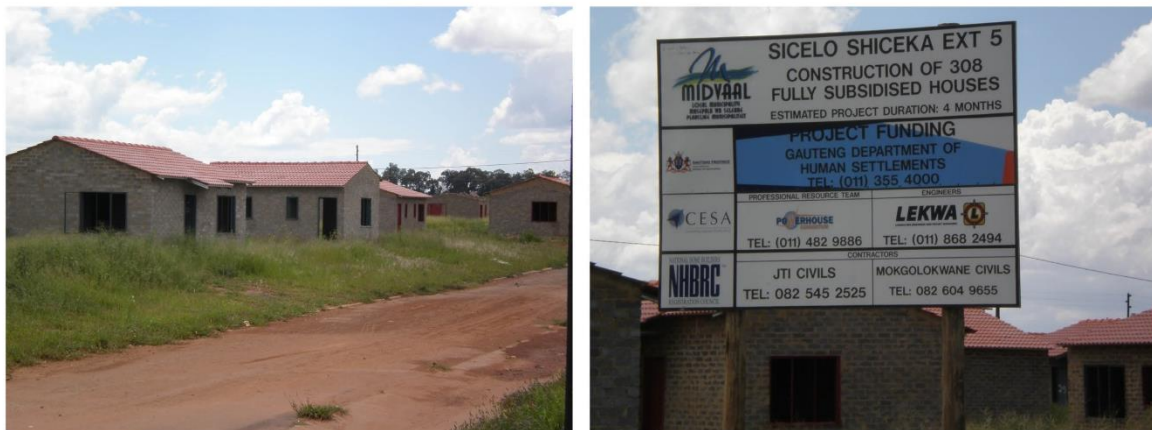
Figure 5.5: The Housing Project in Progress in Sicelo
