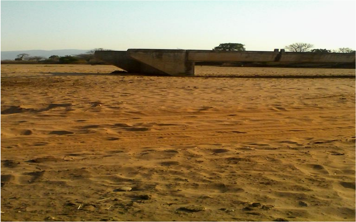
Plate 4.4: Part of Hoya bridge in Muzarabani District Zimbabwe after damage by floods in 2001 to date not yet attended to (2017)
