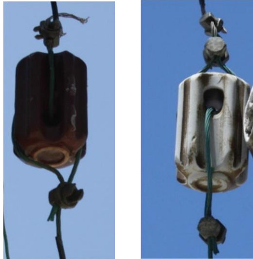
Figure 1.6: Glazed (left) and unglazed (right) downwire (stay wire) insulators [9]
