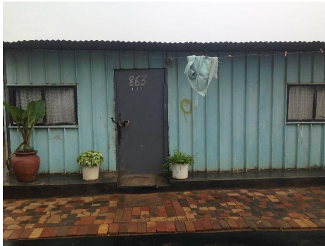
(Margret's Shack. Source, Mohale, N 2017-01-10, N12 Highway Park)
