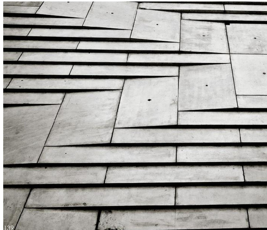
Figure 139: A ramp / stair combo in Leuven, Belgium. M Museum. Architect: Stephane Beel.
