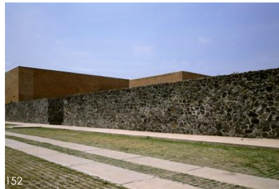
Figure 152 - 155 : The Centre for the Blind and Visually Impaired. A blind wall along the edge of the complex acting as an acoustic barrier and water channels which guide users through the plaza by means of the sound of water.
