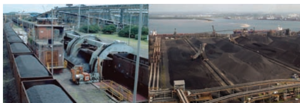
Figure 13—(a) Coal tipplers transferring coal at Richards Bay before (b) being stacked on blending stockpiles
