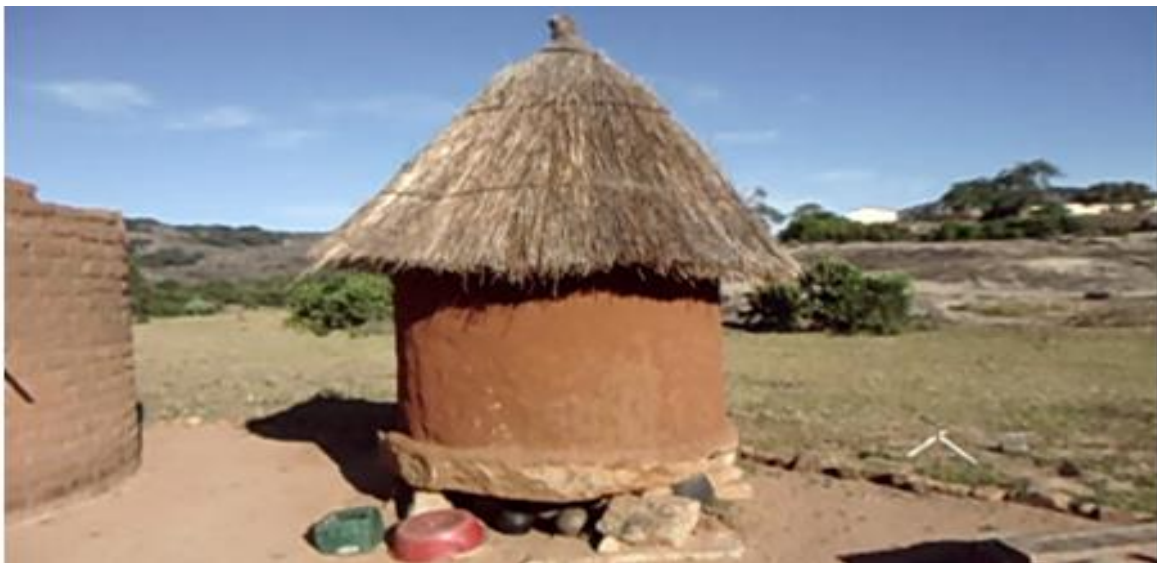
Picture 9b: ‘Hwikwiyo’ with a grass thatched roof supported on a circular base
