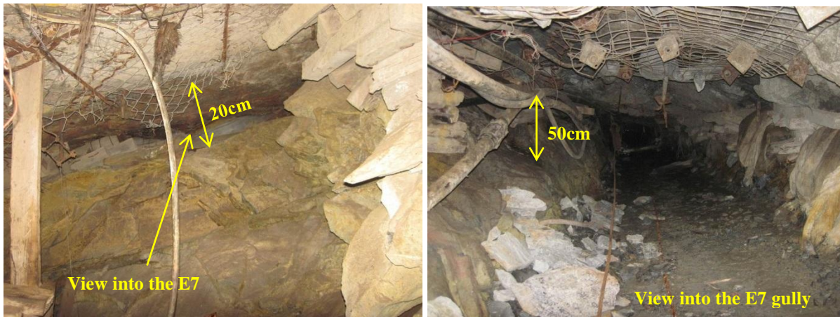
Figure 33. View into E7 stope from the E7 cleaning gully and view of the E7 gully.
