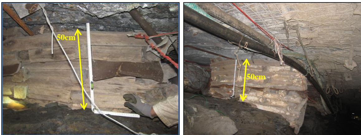
Figure 28. Closure observed on timber pack in the 104-65 W9 cleaning gully.
