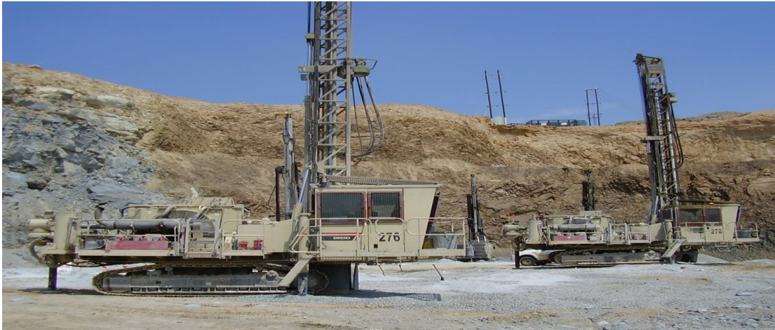
Figure 3. Drill rig use in Opencast mining production pit (Source: https://eureka.angloamerican.com )
