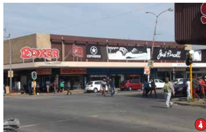
FIG. 108: Photo taken on the corner of Union Street and Beaconsfield Avenue. Photo: author's own
