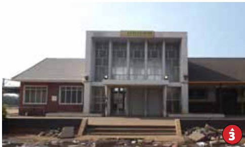
FIG. 96: Main Train Station entrance. Photo: author's own
