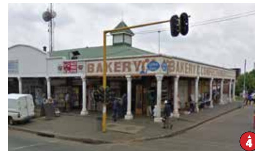
FIG. 125: The Taxido Junction Arcade, corner of Union Street & Beaconsfield Avenue. Photo: author's own
