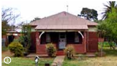
1935 - Type P95A for station Foremen, guards, gangers, pumpers, firemen & shunters. Photo: authors own
