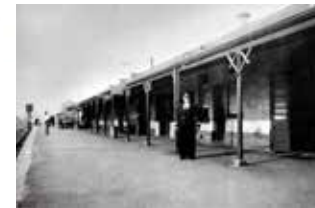
A photo of the Vereeniging Station goods shed (rebuilt after the original was burnt down in 1900) and shortly before the demolition of 1953 (Vaal Teknorama Archives)
