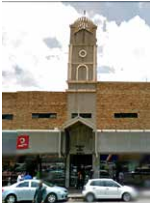
FIG. 32: Vereeniging Jumah Masjid Street elevation Photo: Google earth
