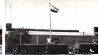
1905 (demolished) Jail built by Dr. Thomas Leslie
