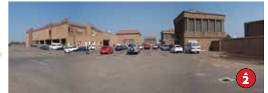
FIG. 70: Markpark Mall roof top parking is isolated from the rest of the city, which the ramp being the only access. Walls measure approximately 2.3m high and are impossible to look over. Photo: author's own
