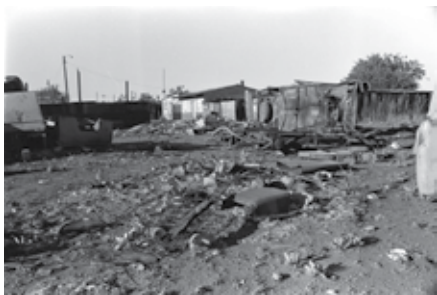
1959 Demolition of Top Location. Photo: Yusif Gathoo
