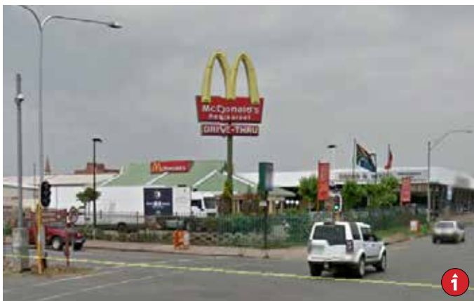
FIG. 105: The McDonalds drive-thru on the corner of Voortrekker Street and Rhodes Avenue. Source: Google earth
