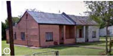
1894 - NZASM row housing, this preserved example is similar to ones found in Germiston & Boksburg. Photo: authors own
