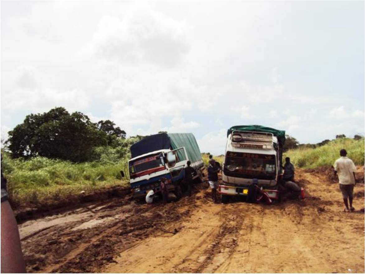
Figure 3.3: Tanzania unpaved roads condition during rainy season (Source: Michuzi Blog 2010)
