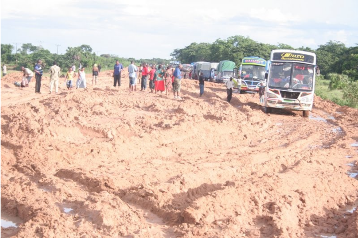
Figure 3.4: Tanzania unpaved roads condition during rainy season (Source: Michuzi Blog, January, 2013 at Lindi-Mtwara road)
