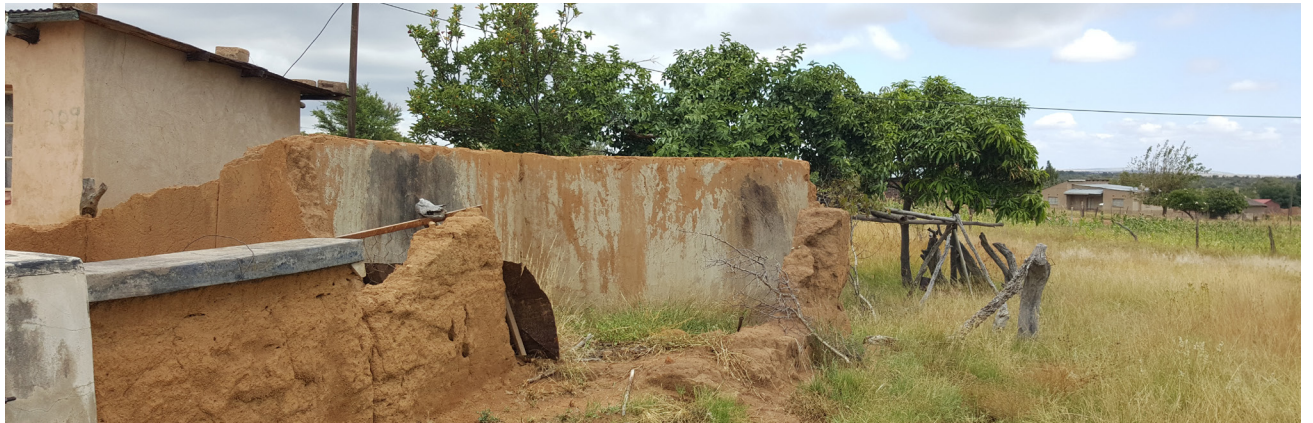
The old kitchen tied to the perimeter wall position.
