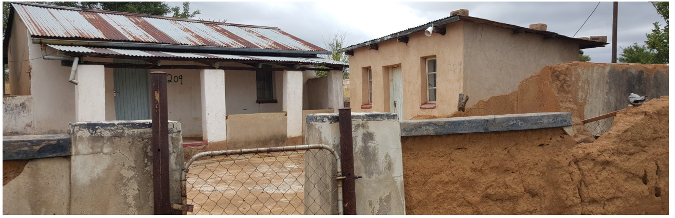
The walls enclosing the lapa were built of daub and covered with store bought copings to prevent rain from ruining them prematurely, with the ruins of the old kitchen hut joined to the entrance wall.
