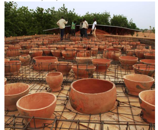
Figure 3.37b. – The pots were used as moulds on the roof, for natural light to enter the roof into the library.
