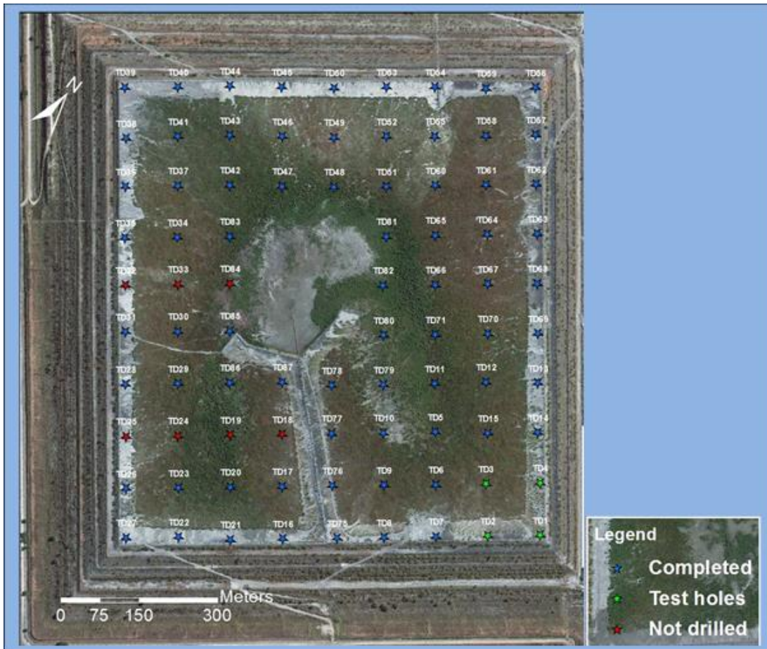
Figure 6: Aerial view of the Case Study tailings dam
