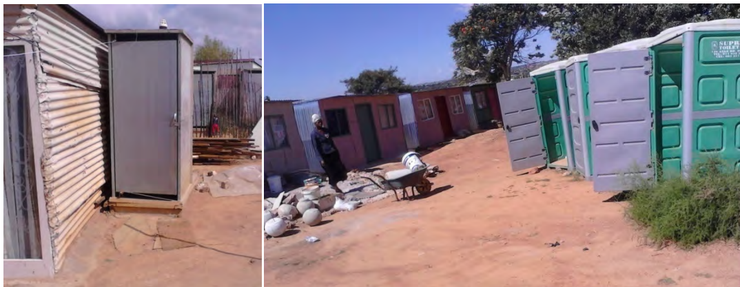
Figure 6.5. Toilets used in Ruimsig Informal settlement: earlier supplied VIP toilets –left; more recently supplied chemical toilets - right. Source: Author’s Photographs, 2015.
