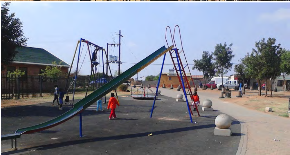
Figure 7.9 Three of the ten existing parks in Cosmo City Source: Author's Photographs, 2014.
