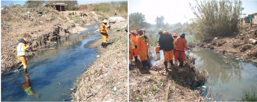
Figure 5.18. EPWP workers cleaning the Northriding stream in Kya Sands settlement.
