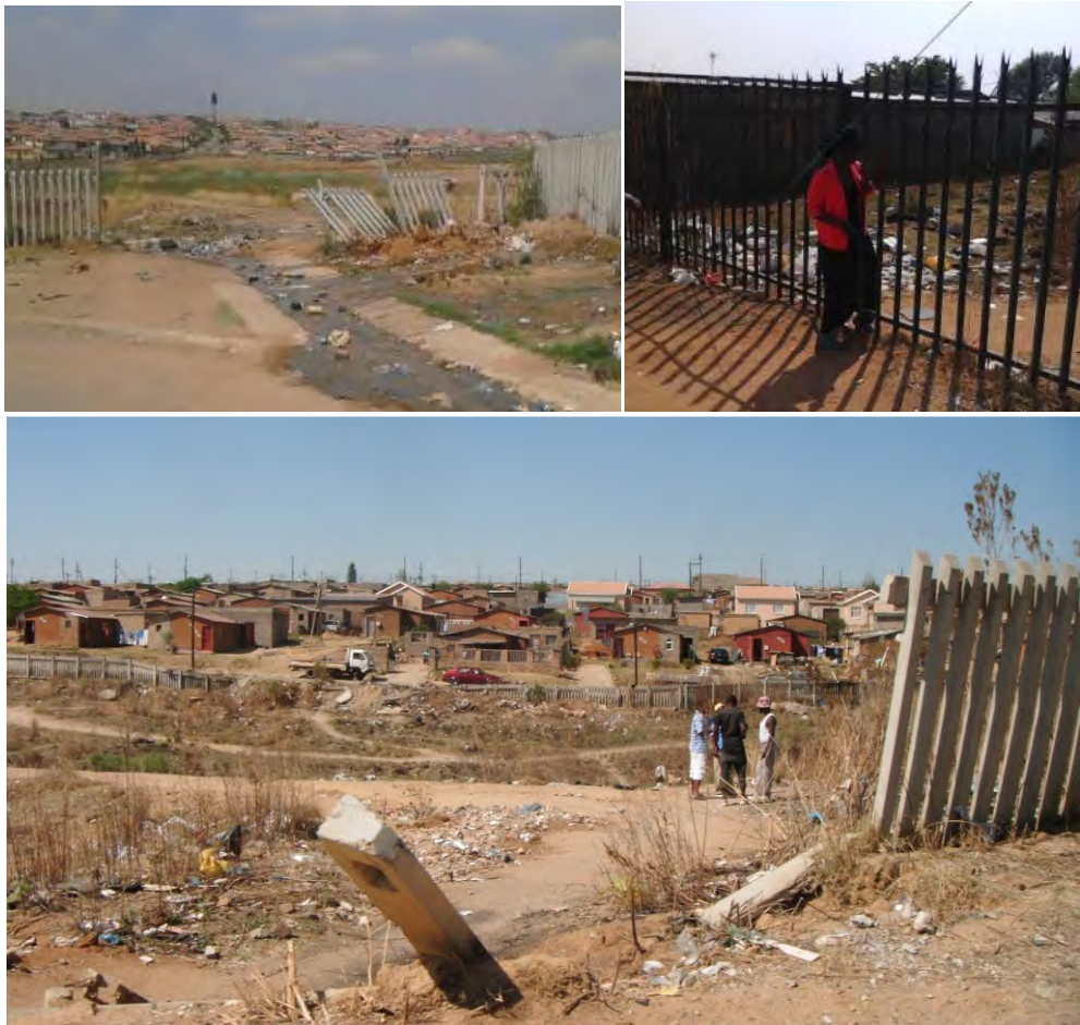
Figure 7.10. Broken palisades fencing at different points around the Green Belt in Cosmo City.
