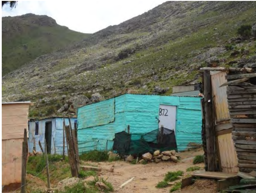
Figure 2.2 Langrung informal settlement in Stellenbosch (Western Cape, South Africa) is located on a steep hillside Source: Author's Photograph, October 2013.
