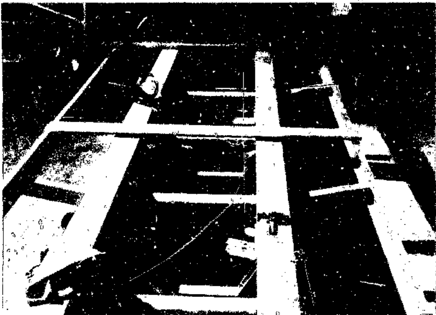
Photograph 5.27 Side rails positioned and tacked to outriggers
