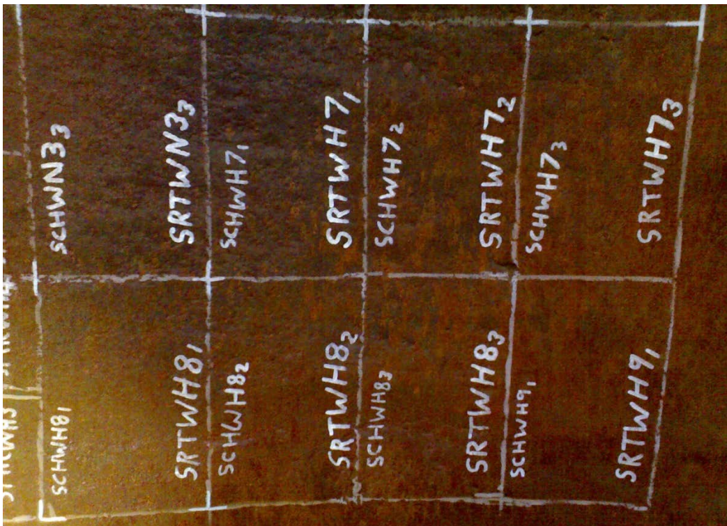
Figure 3.2: Representative photograph showing sample areas as marked out on the shell of the ash lock.
