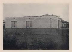
6. Wall plate anchored to wall, but trusses and roof removed
