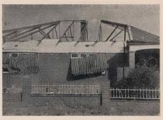
7. Trusses anchored to wall but purlins and raofing removed.
