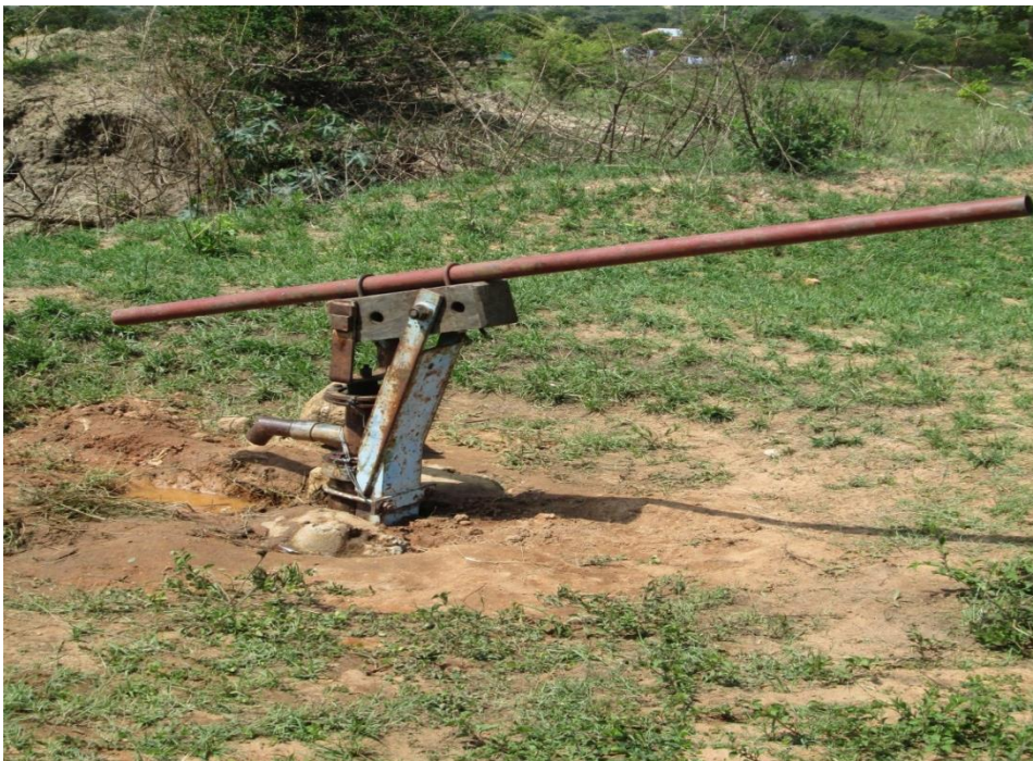
The only borehole in the village
